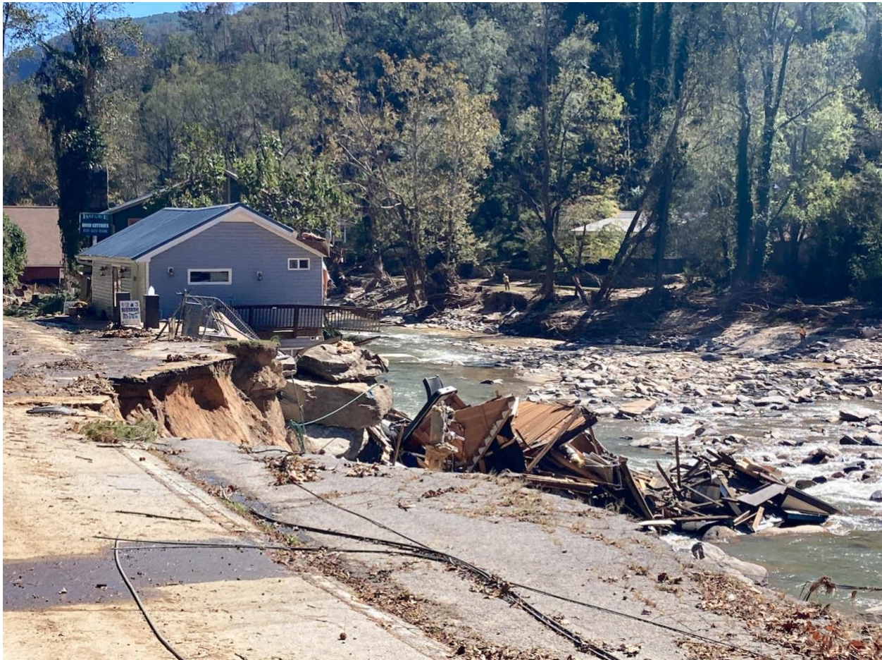
Figure 11: Flood Damage along US Route 64, Bat Cave, NC, October 10, 2024. Credit: NCDOT
