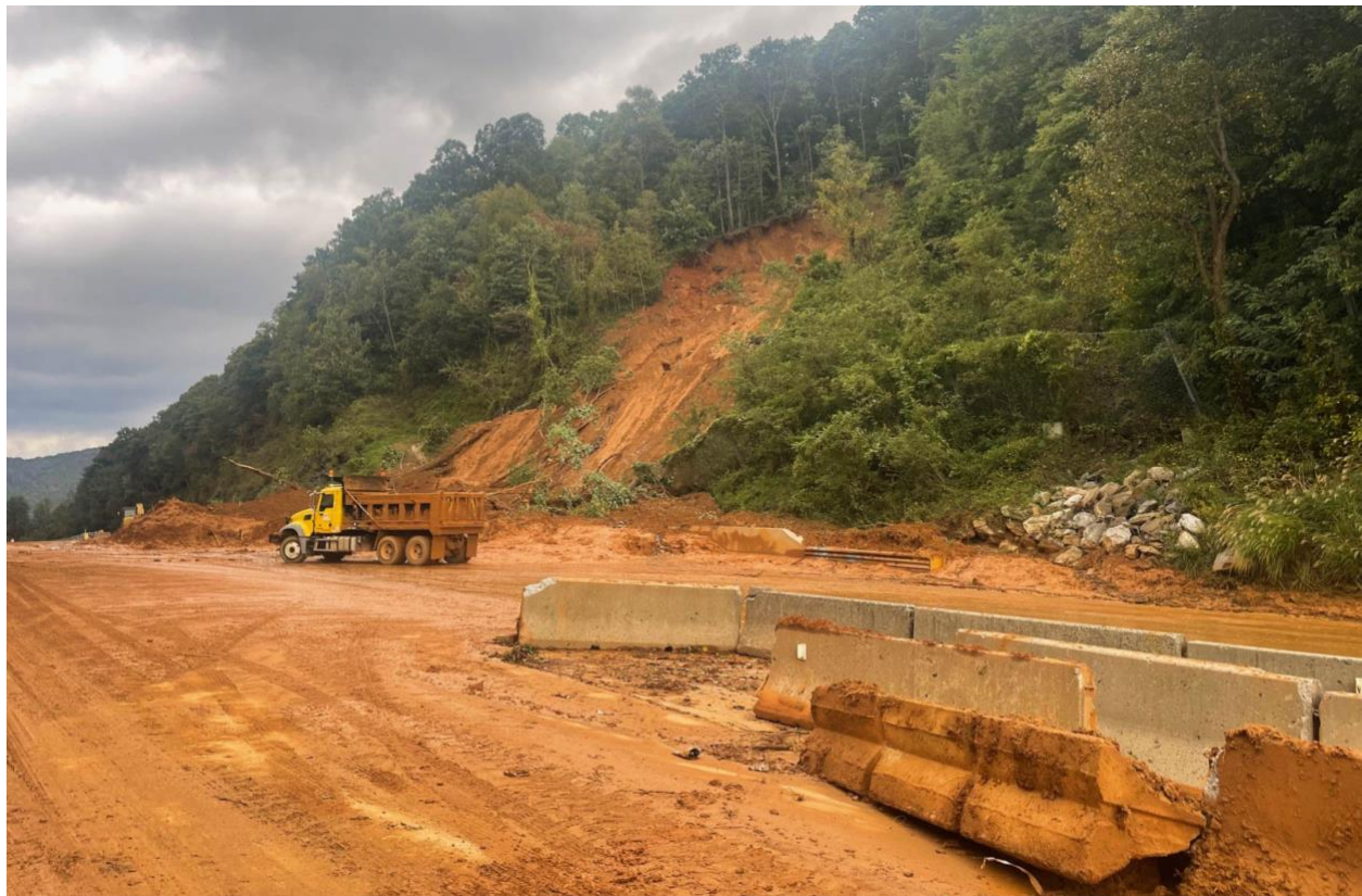
Figure 10: Aftermath of Helene-Triggered Mudslide, September 28, 2024 (Credit: NCDOT)
