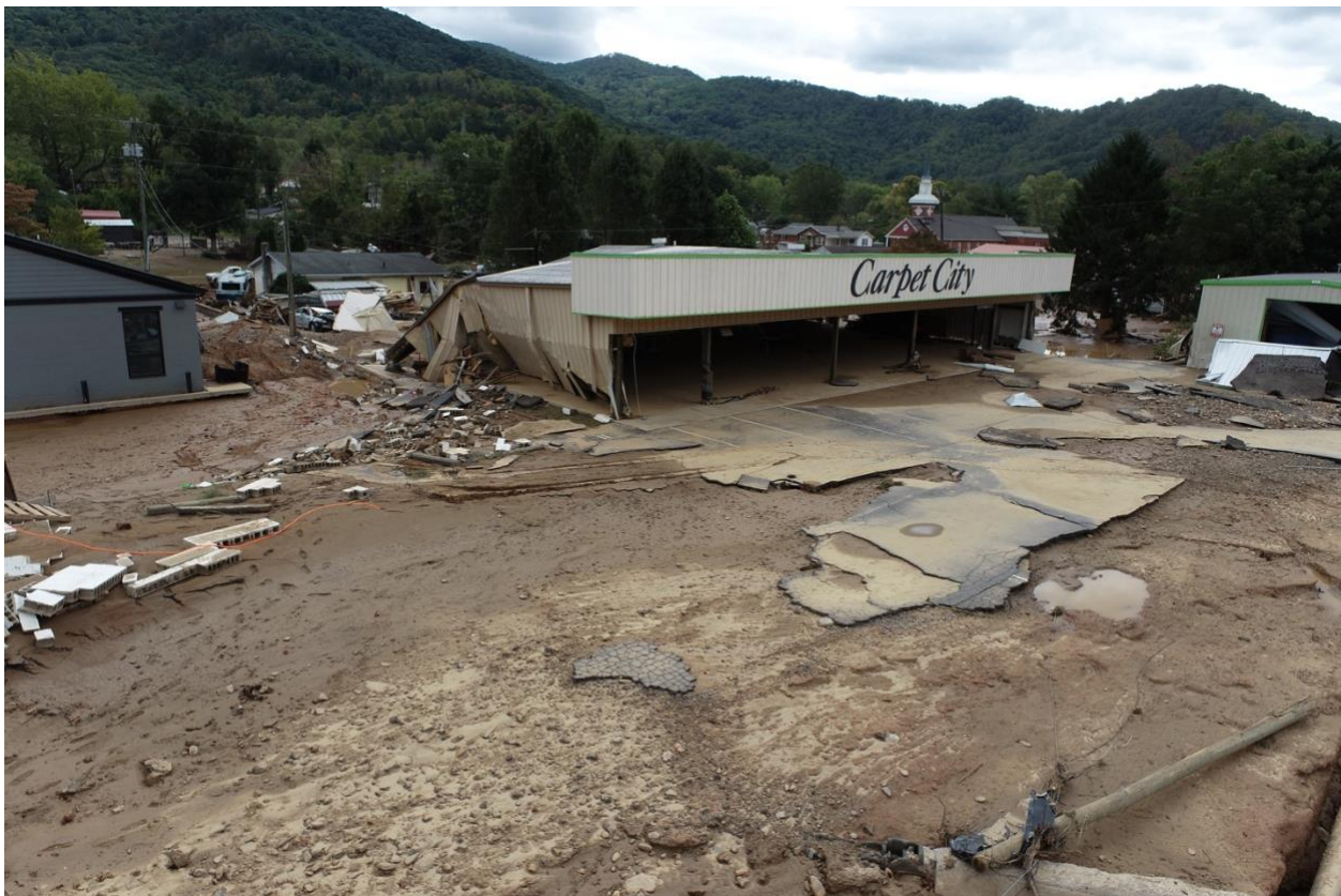
Figure 9: Poverty Branch Road, Madison County, September 29, 2024. Credit: NCDOT.
