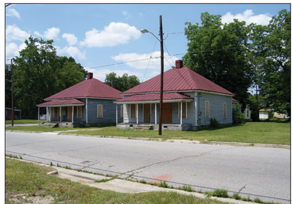
Boarded Up Housing Units in Rocky Mount, NC
