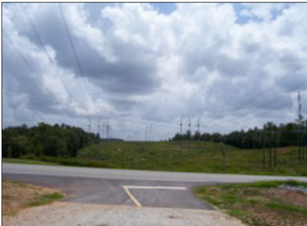
Overhead power lines have caused some concerns about public health but evidence of public health effects are mostly considered inconclusive.
