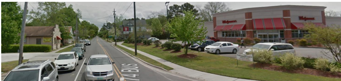
The newer Walgreens drug store and older commercial development along Martin Luther King Jr. Highway looking east.
