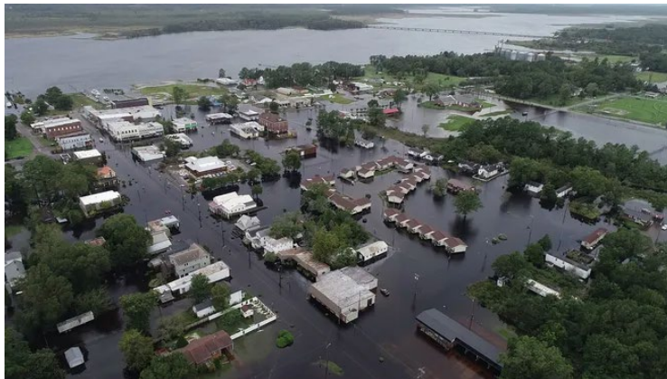
Flooding from Hurricane Florence in 2018 devastated the Town of Belhaven (Beaufort County) Credit: USA Today
