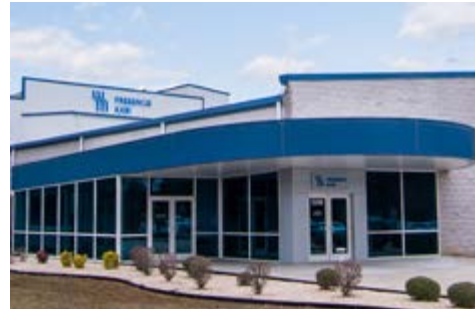
Fresenius Kabi's current facility in Wilson, N.C.
