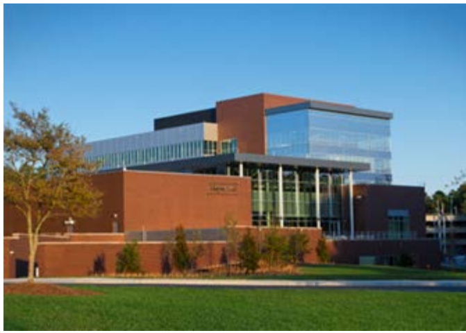
Biogen Idec Building 26 in Research Triangle Park (Photo courtesy of Business Wire)
